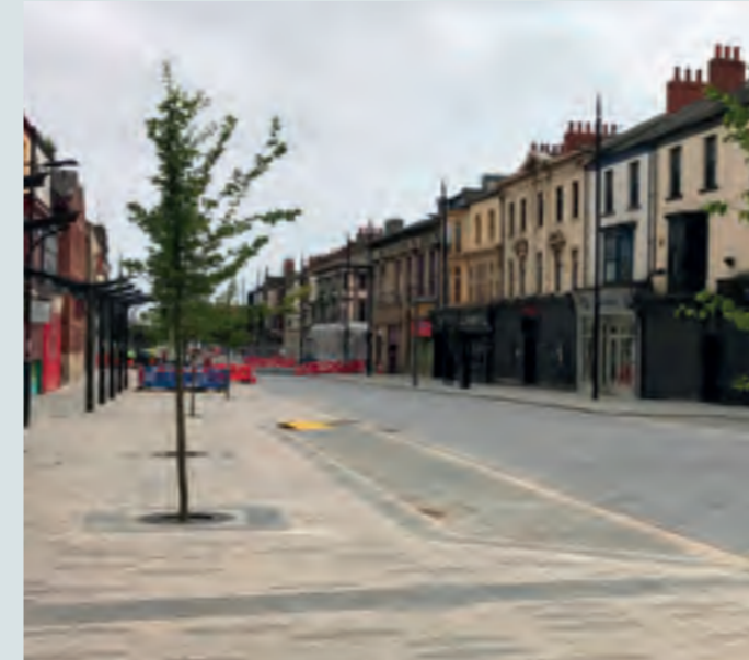
Figure 9: Refurbished Church Street, Hartlepool
