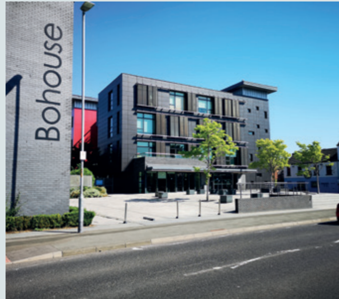
Figure 3: Bohouse, Bridge Street
