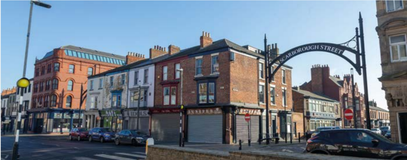
Figure 29: Scarborough Street today
