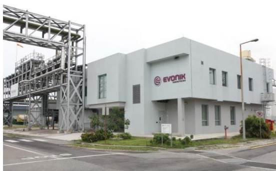
Evonik Industries Singapore. Source: Siemens Pte Ltd
